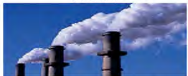
Visualization of fugitive emissions leaks
